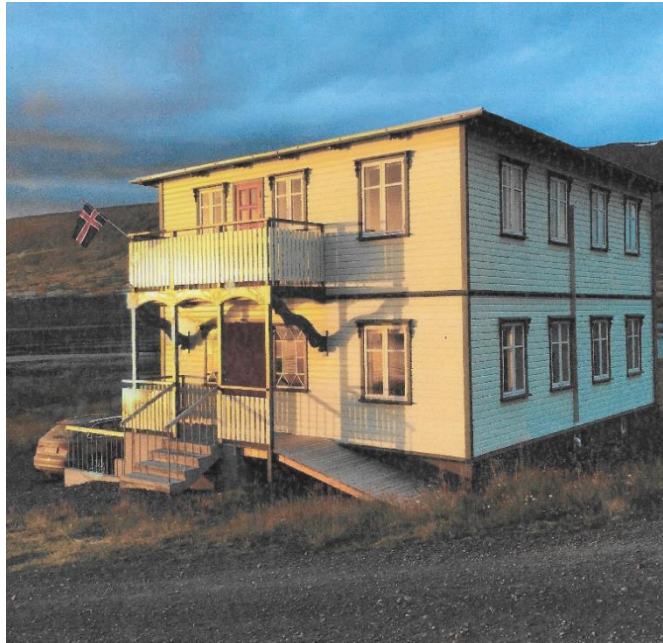
Figure 13: Kolkuos guesthouse after the renovation.
