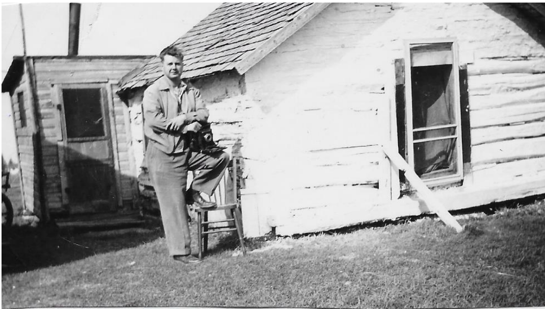
Figure 3: Photograph of Fridjon and Gudny's historic house in Gimli taken by their grandson Robert Harold Frederickson (in picture) in the summer of 1952.
