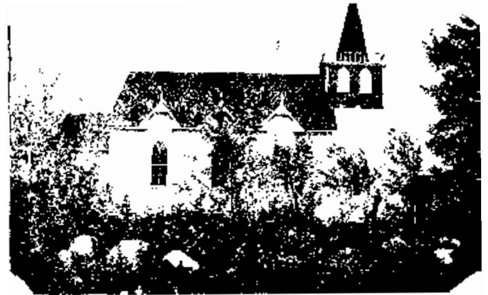
Breiðuvík church, located in the southeast corner of Kirkiubæ
