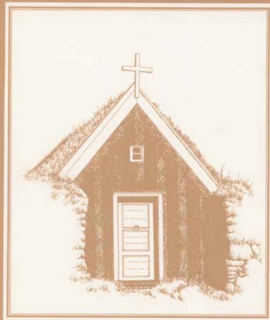
A 17th Century turf-built chapel at Nupsstadur in southern Iceland. The interior of the building is only 6 metres long and 2.5 metres wide. (Drawn by Eric Crone.)
